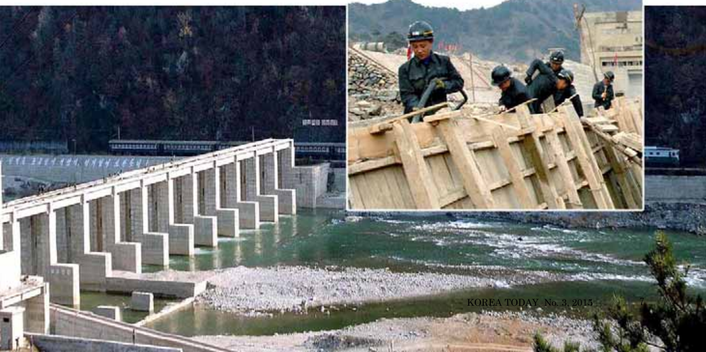
Power stations go up along the Chongchon River.
