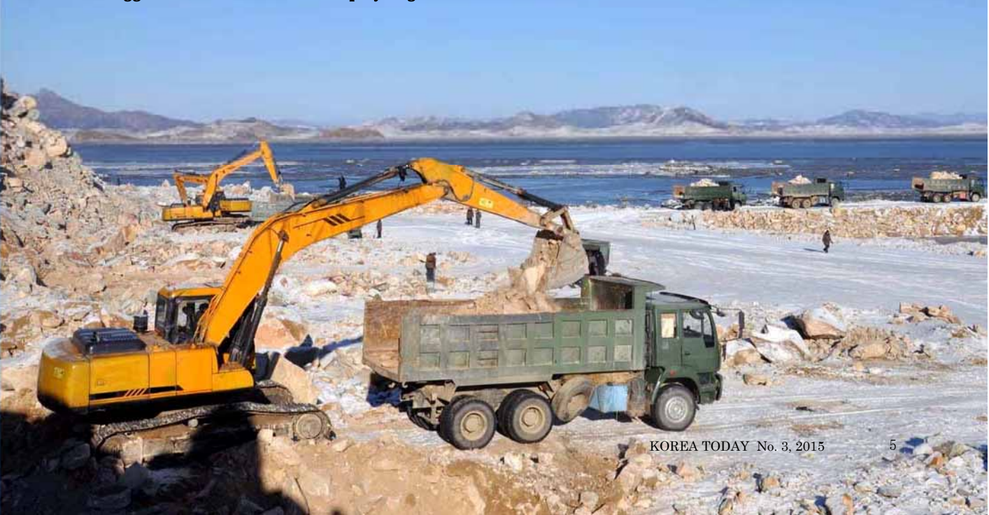
The Honggondo tideland reclamation project goes full steam ahead.
