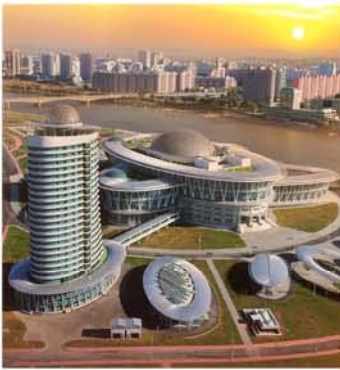
Front Cover: The Sci-tech Complex
