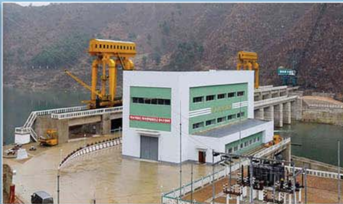
Huichon Power Station No. 4
