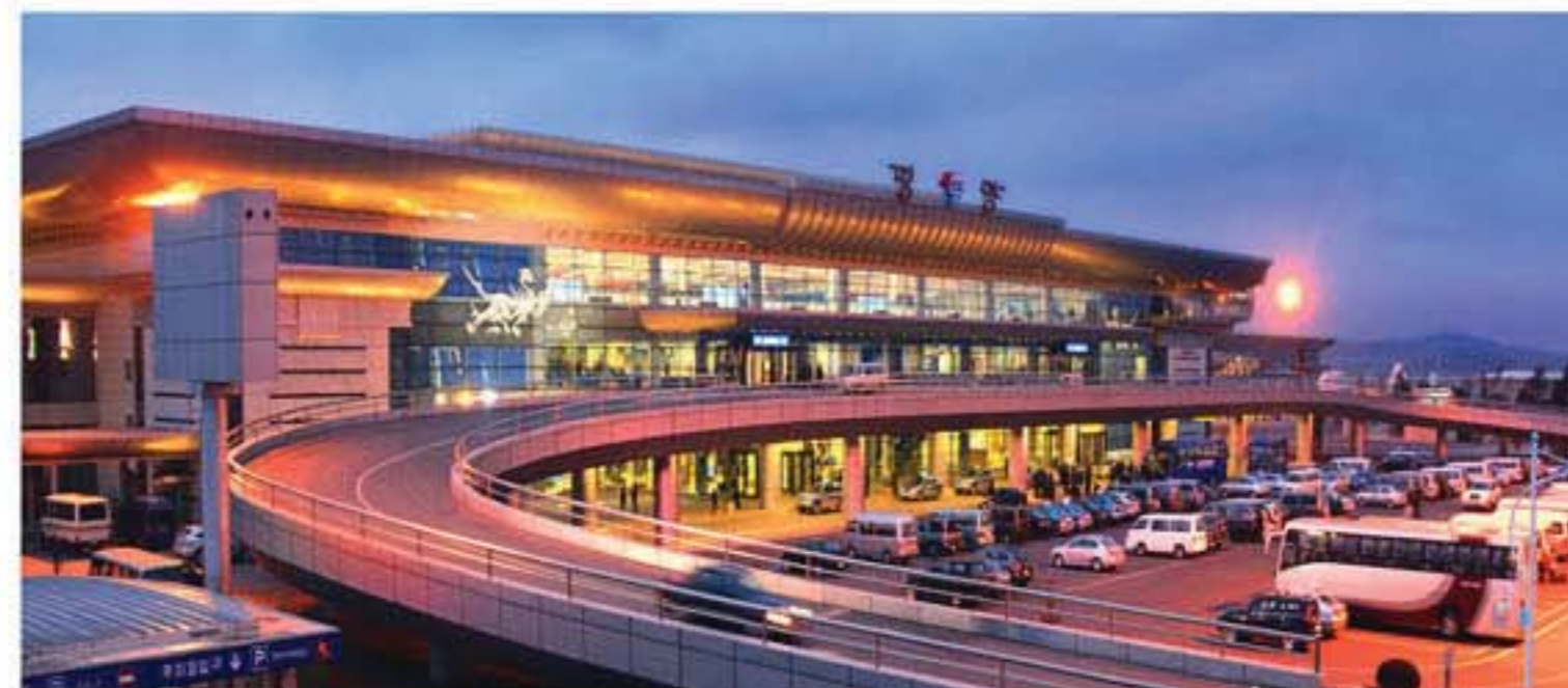
Terminal of Pyongyang International Airport
