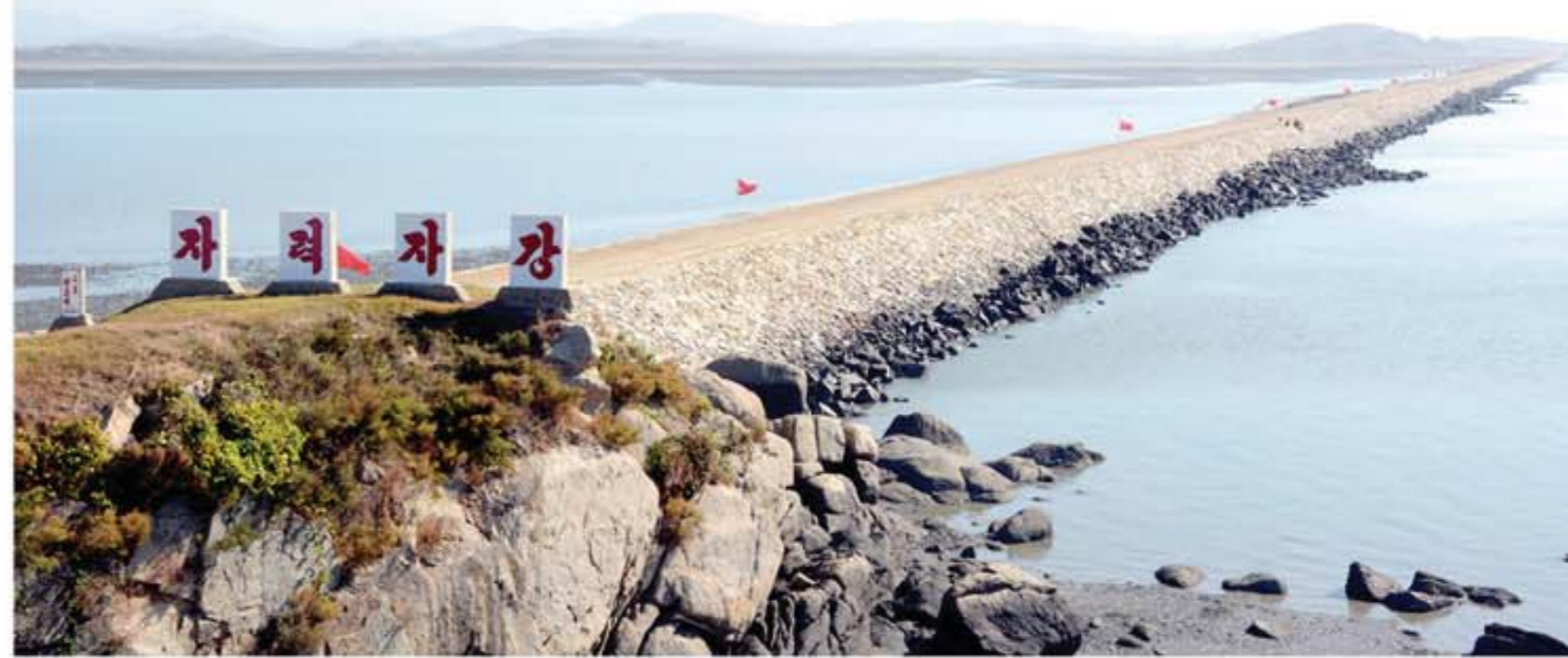
The first-stage construction of the Honggondo Tidal Land was completed.
