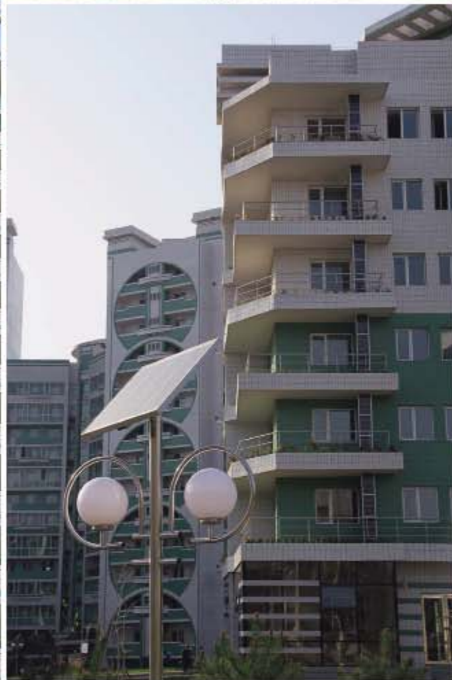
Solar panels and solar water heaters are attached on the walls of the apartment buildings and to lamp posts, and installed on the rooftops of the public buildings in order to make effective use of natural energy resources
