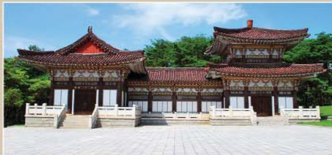
External view of the hall for memorial services
