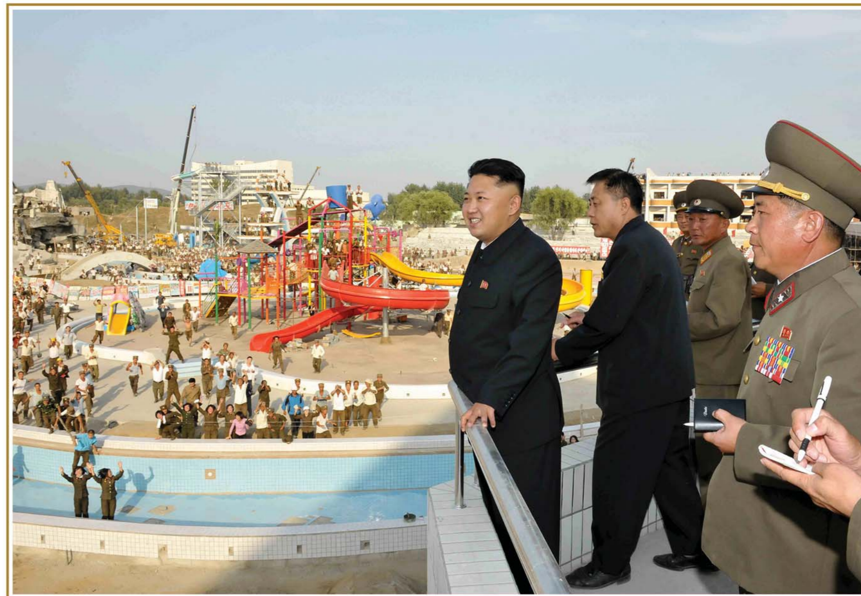
Supreme Leader Kim Jong Un visiting the construction site of the Munsu Water Park [September Juche 102 (2013)]
