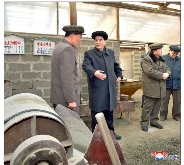
Premier Pak Pong Ju (second from left) on an inspection tour of the renovation project for Samjiyon County.
