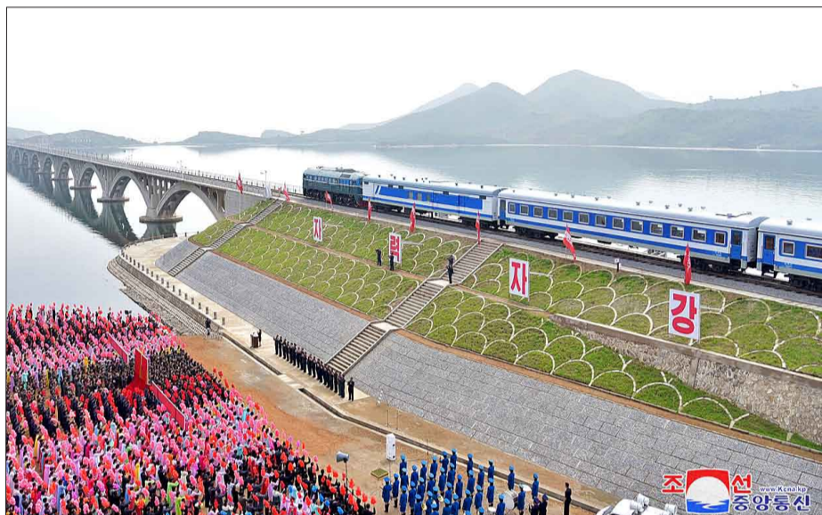
The new railway links Koam and Tapchon in Sokjon Bay.
