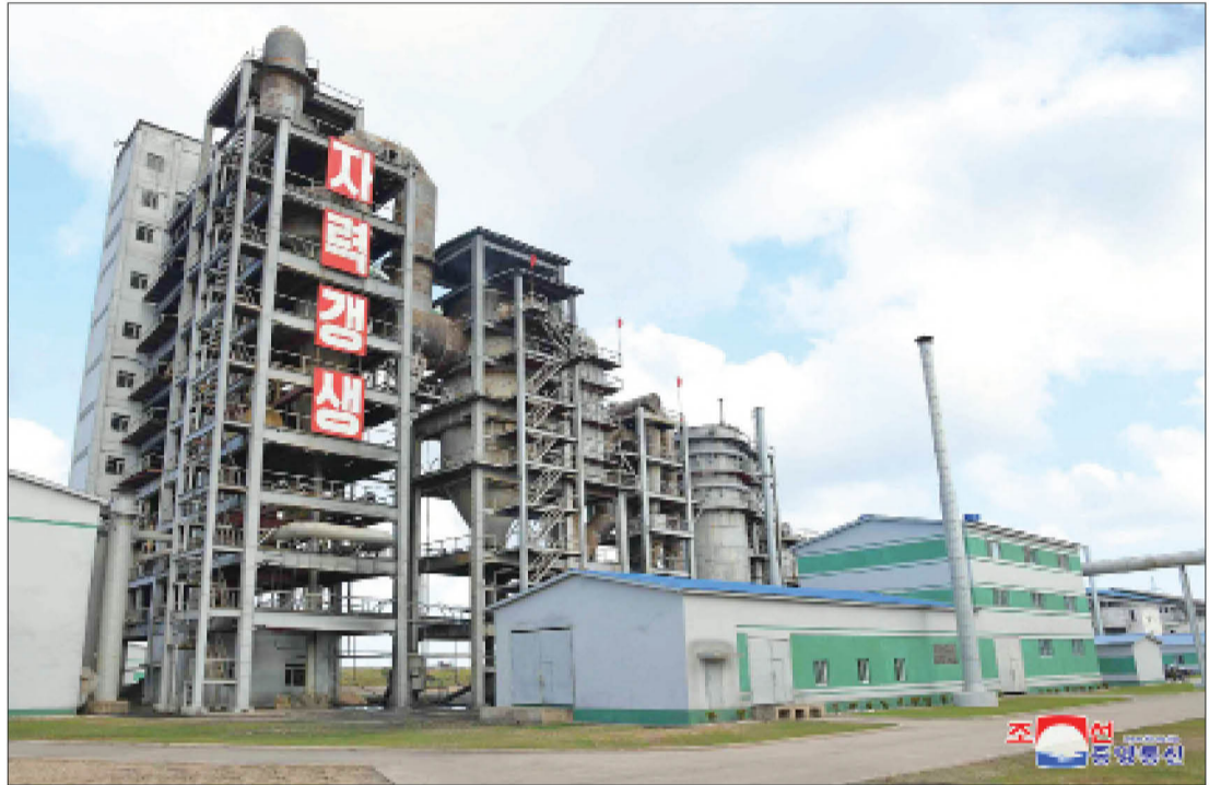
The Kim Chaek Iron and Steel Complex has completed a coke-free production process that includes an oxygen blast furnace.
