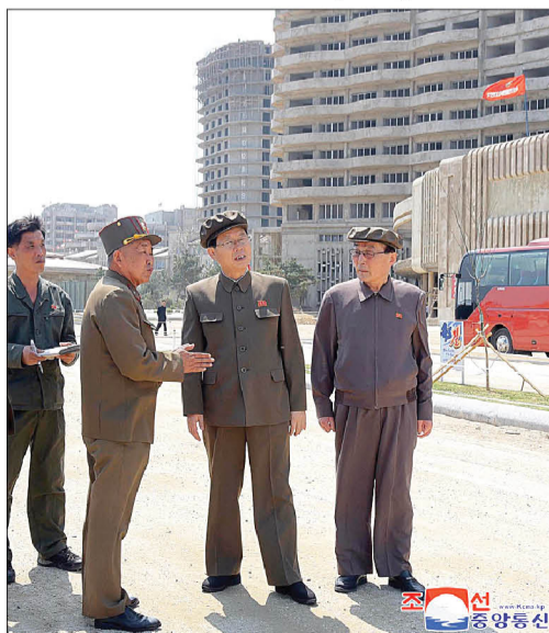
Premier Kim Jae Ryong (second from right) visits the construction site of the Wonsan-Kalma coastal tourist area.
