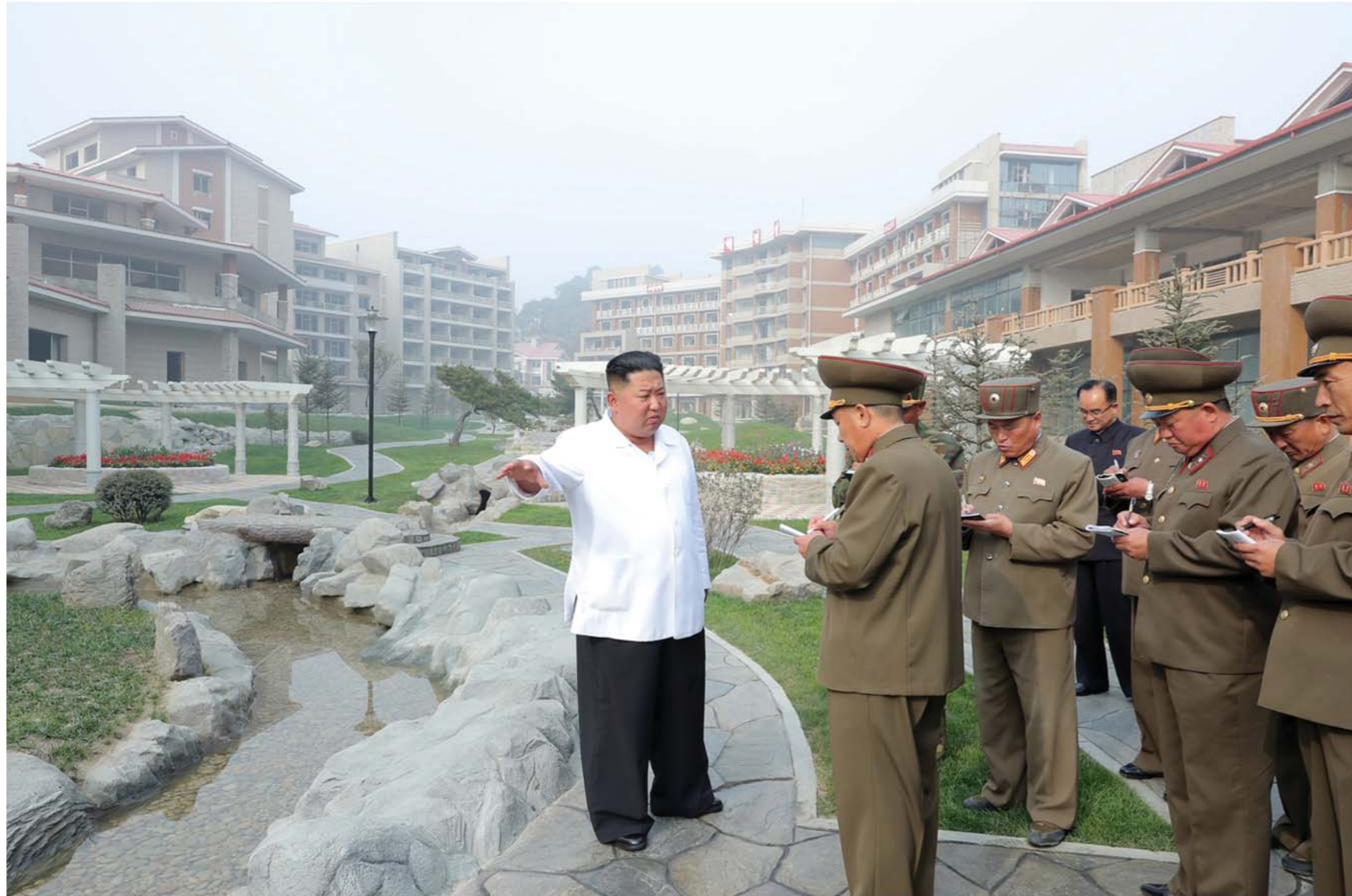
The Supreme Leader gives field guidance at the construction site of the Yangdok County hot spring resort that nears completion
