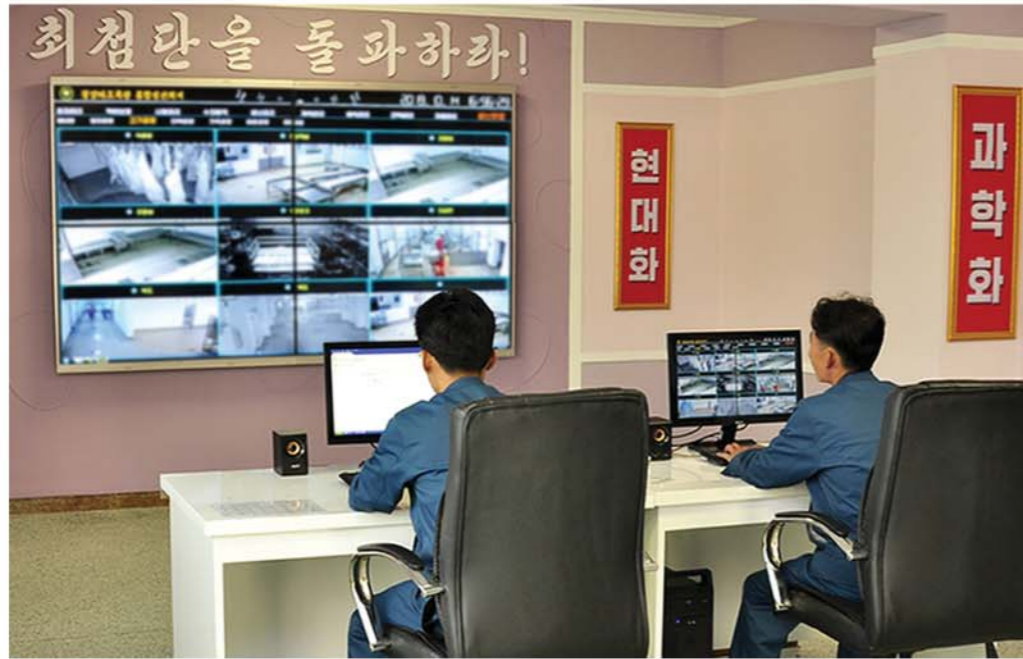
General control room
