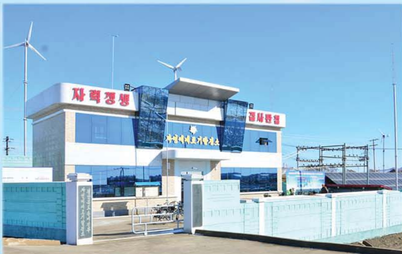
A renewable energy power plant.
