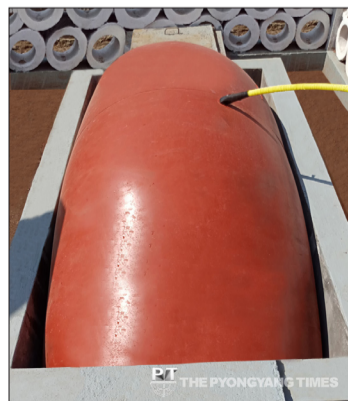
JON KWANG HUN Methane gas tank made of flexible polyvinyl chloride resin for family use.
