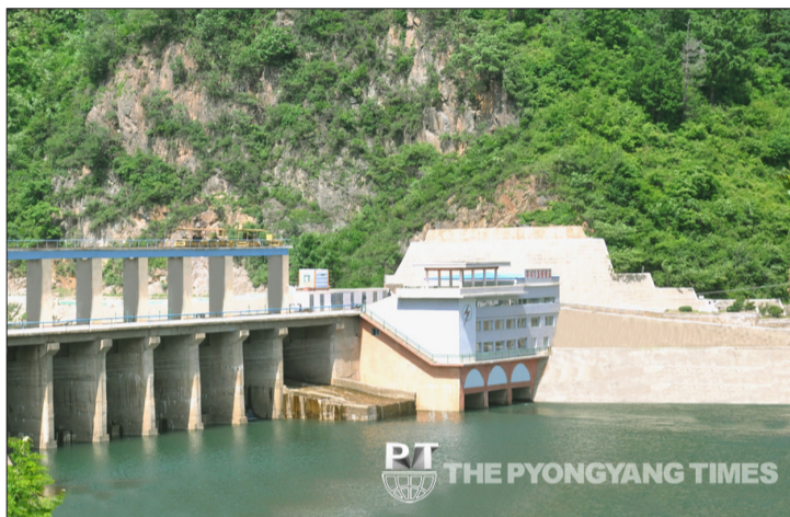
Usi Power Station Unit 1 in Jagang Province supplies power to local factories and residential quarters.
