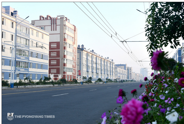
A partial view of the refurbished street in Nampho.
