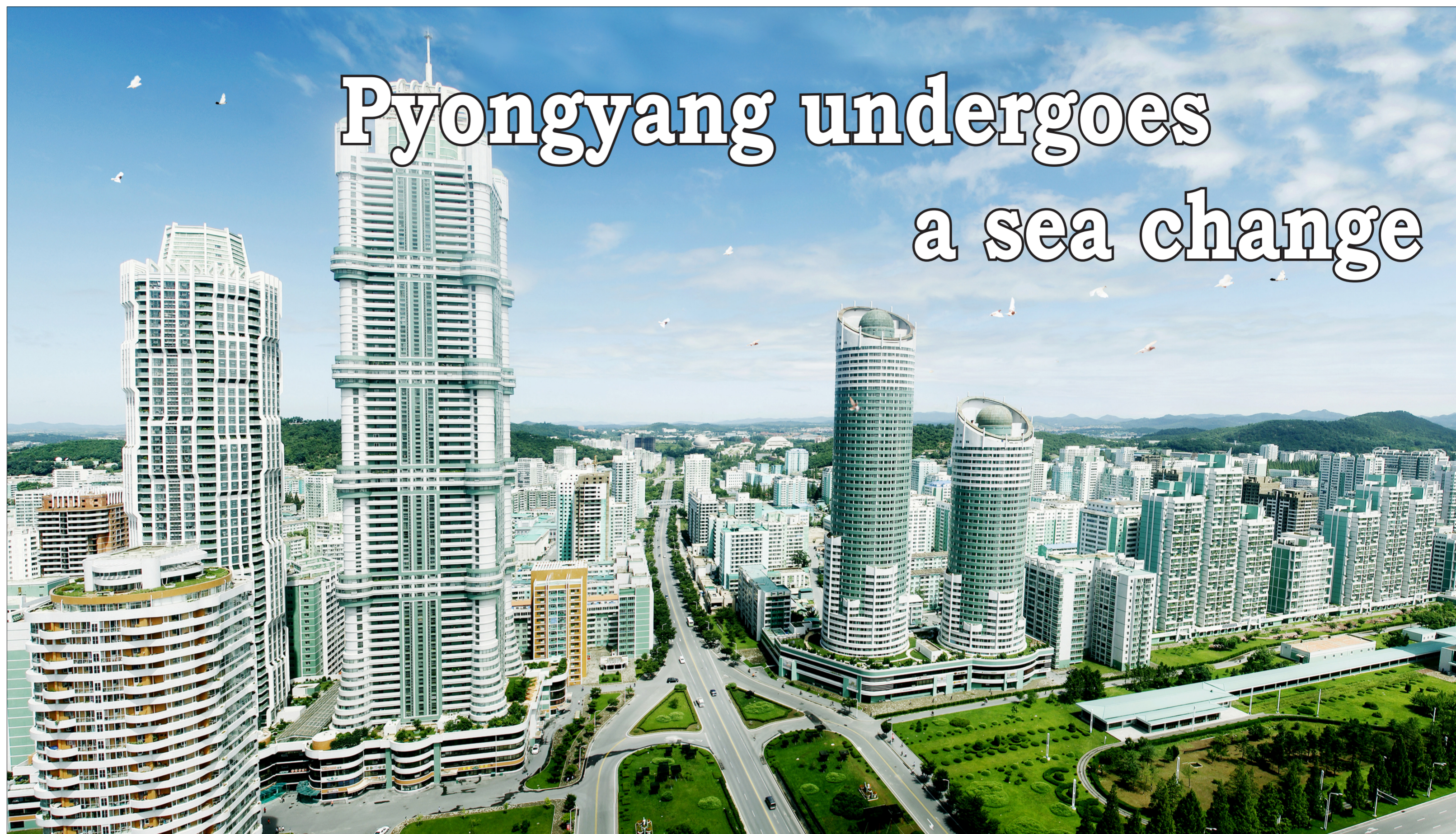
An aerial view of Ryomyong Street, an energy-saving and green one.
