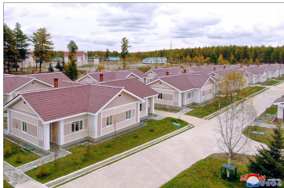
Newly built dwelling houses in Samjiyon, a sacred place of the Korean revolution.
