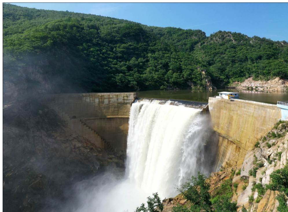
Orangchon Power Station Unit 3 is completed on August 4.
