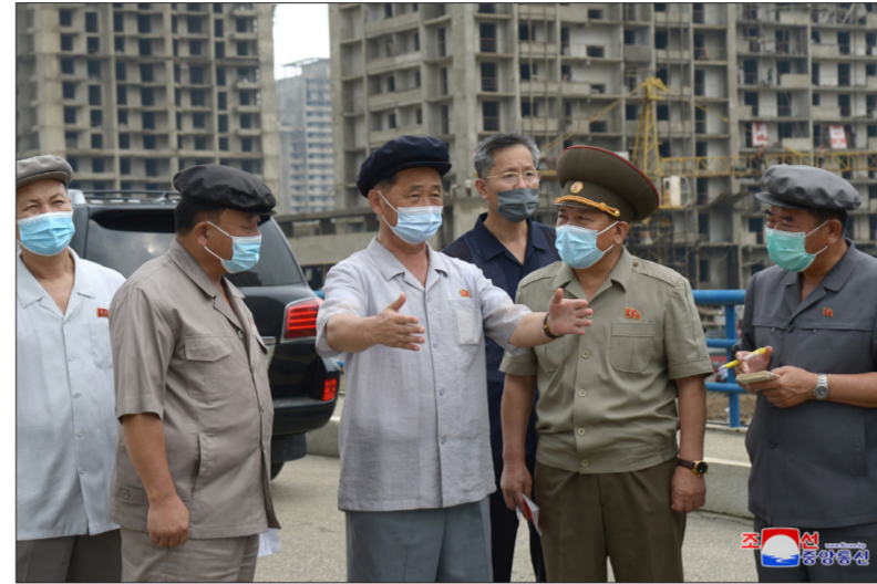
Premier Kim Tok Hun (third from left) inspects the construction site of 10 000 flats in the Hwasong area.
