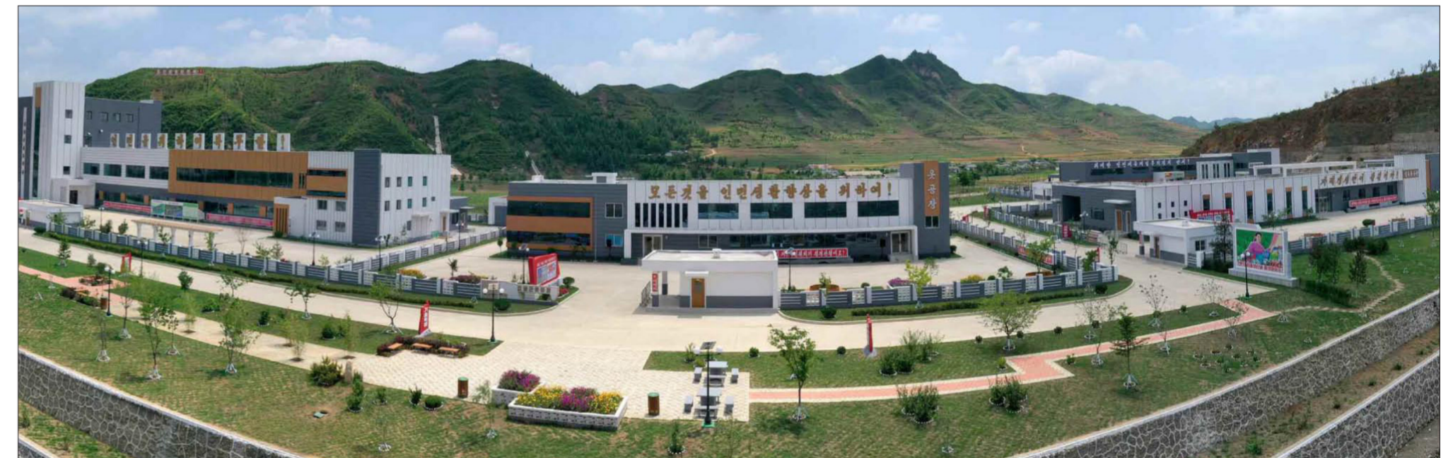
Facelifted local industry factories in Kimhwa County of Kangwon Province.
