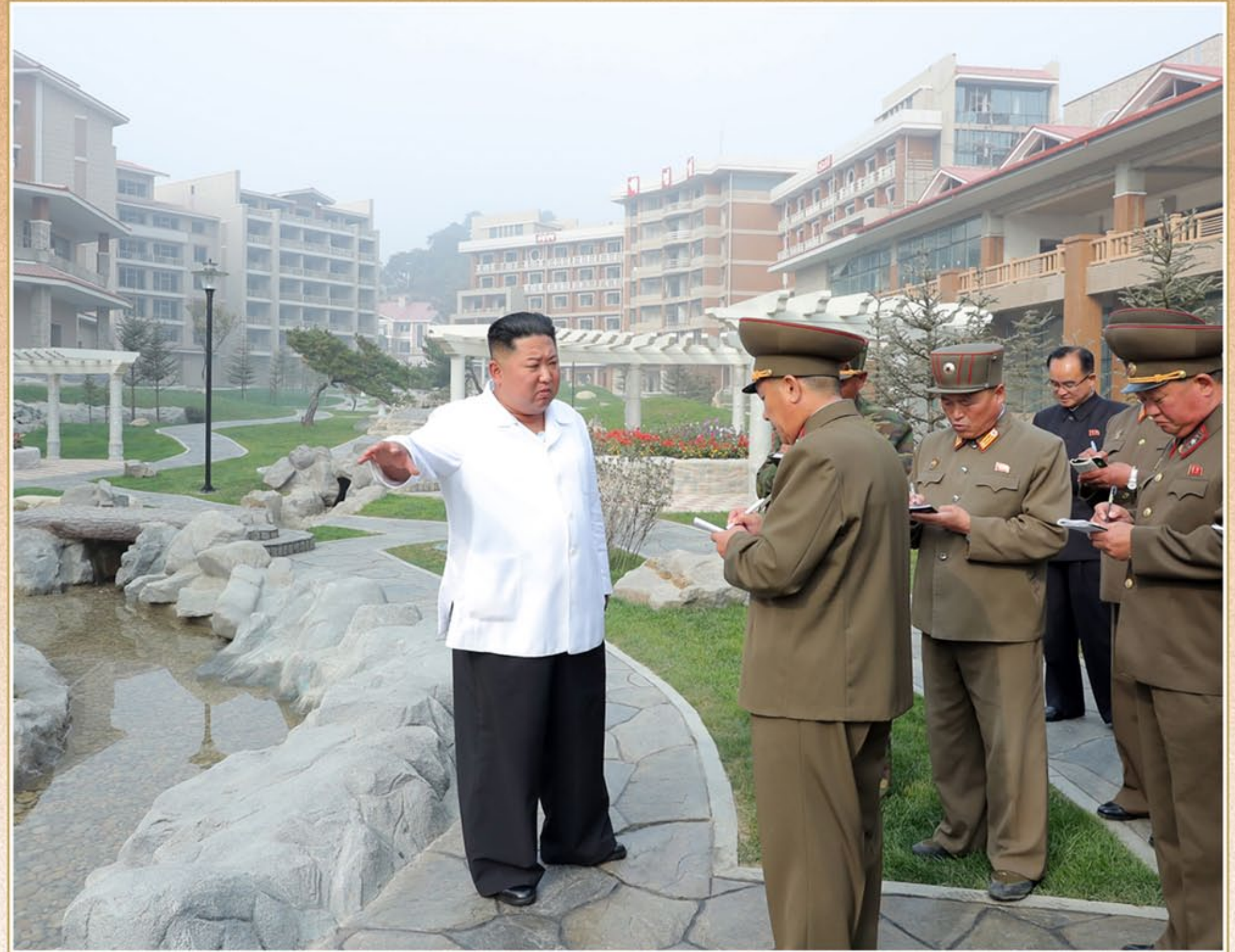
Kim Jong Un inspecting the construction site of Yangdok Hot Spring Resort nearing completion (October 2019)
