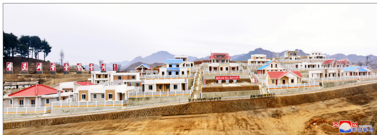
House-moving takes place at the Jasan Farm, Phyongsong City (top left), the Sosin Vegetable Farm in Ryokpho District, Pyongyang (top right) and the Ryonghung Farm in Thaecheon County, North Phyongan Province (above).
