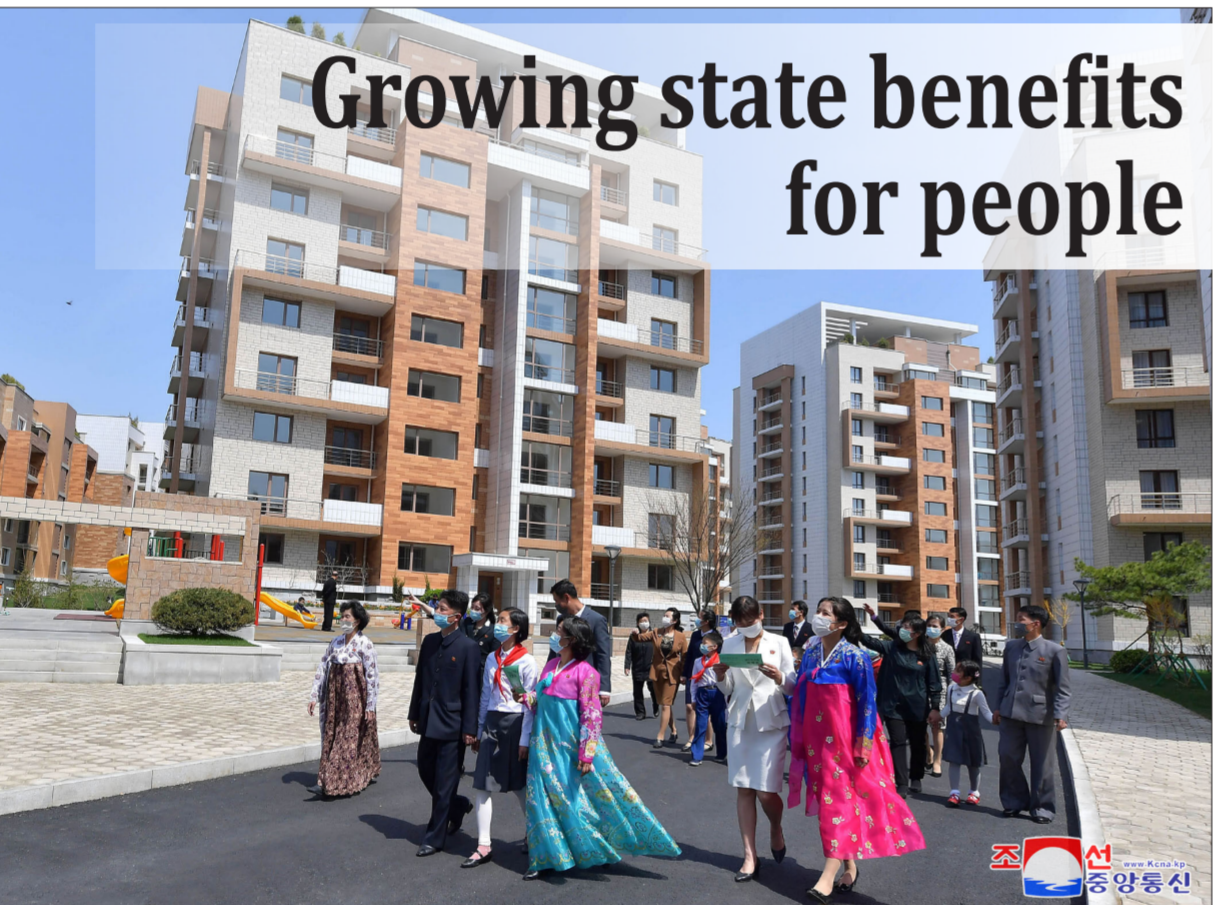
Labour innovators and merited persons move into luxury houses in Kyongru-dong, Central District, Pyongyang.
