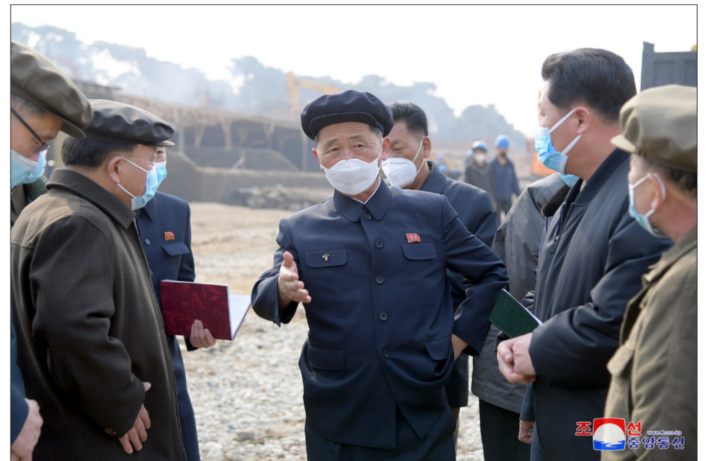
Premier Kim Tok Hun (centre) inspects the construction site of a new street in the Sopho area of Pyongyang.
