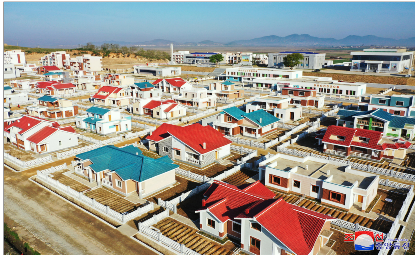
Modern farmhouses are built in many rural villages across the country.
