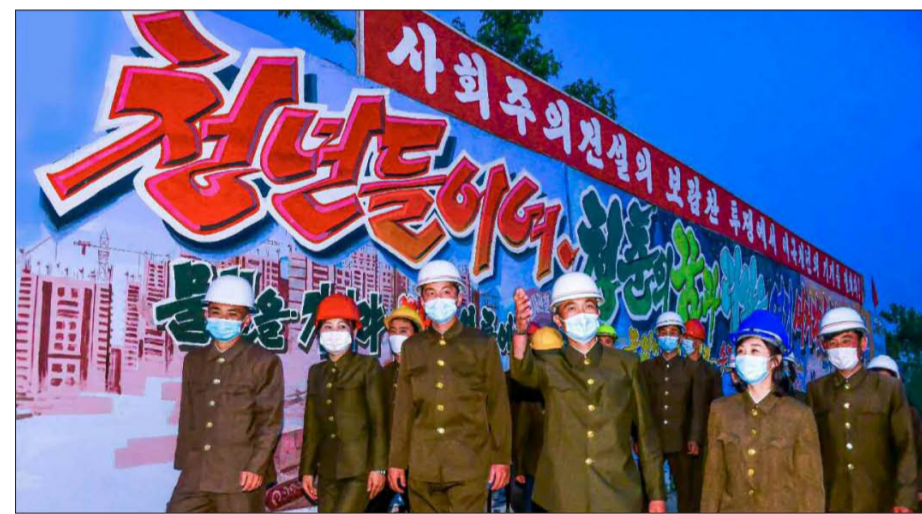
Young people offer night assistance at the construction sites of the capital city. RODONG SINMUN
