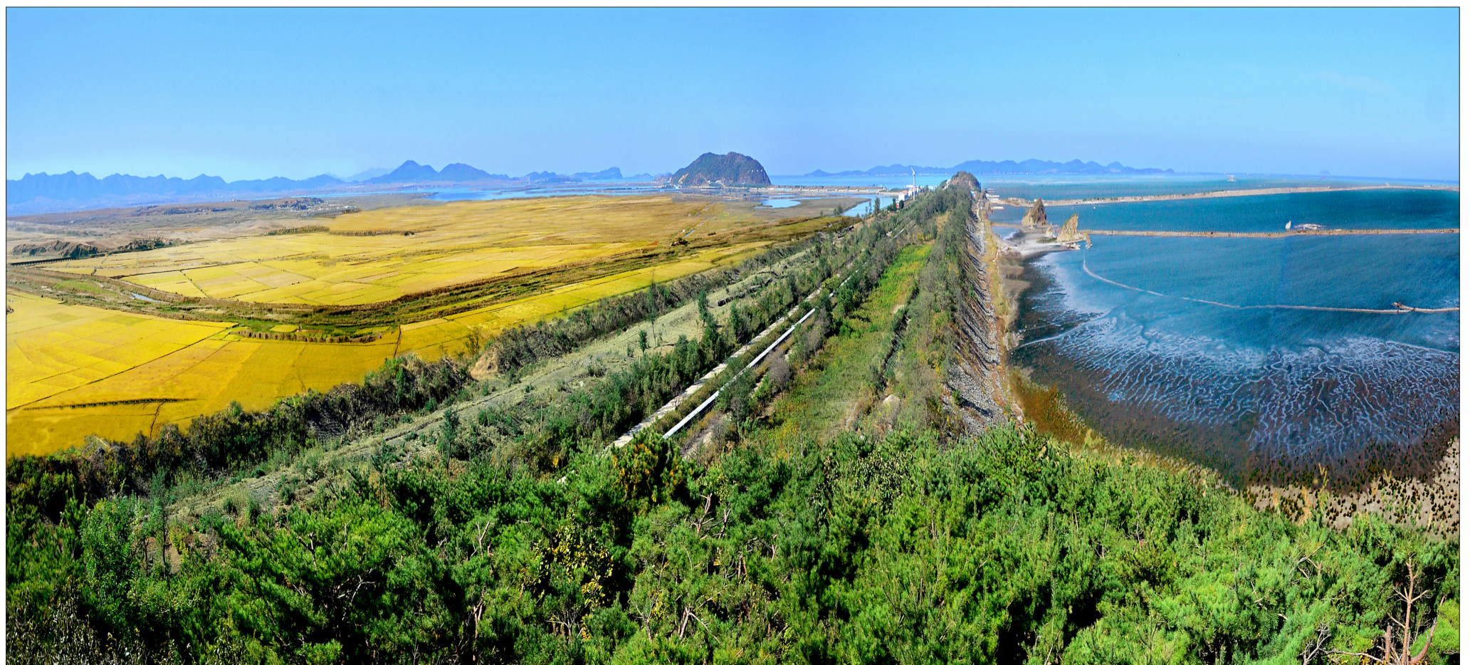
New farmland is increased by damming the sea with overburden brought by the long-distance conveyor belt. RYU KWANG HYOK / THE PYONGYANG TIMES
