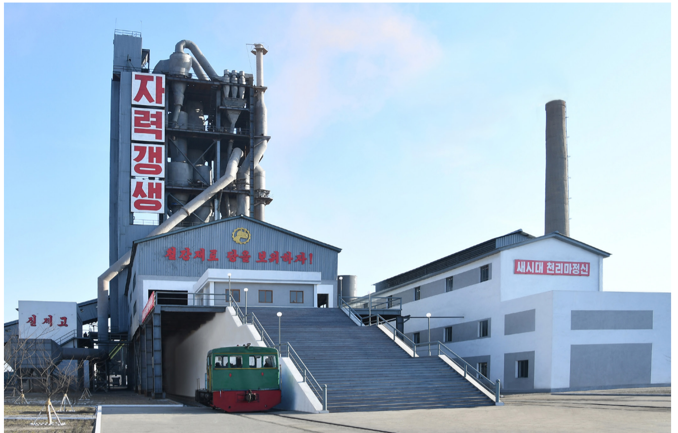
A Korean-style energy-saving oxygen blast furnace built at the Hwanghae Iron and Steel Complex.
